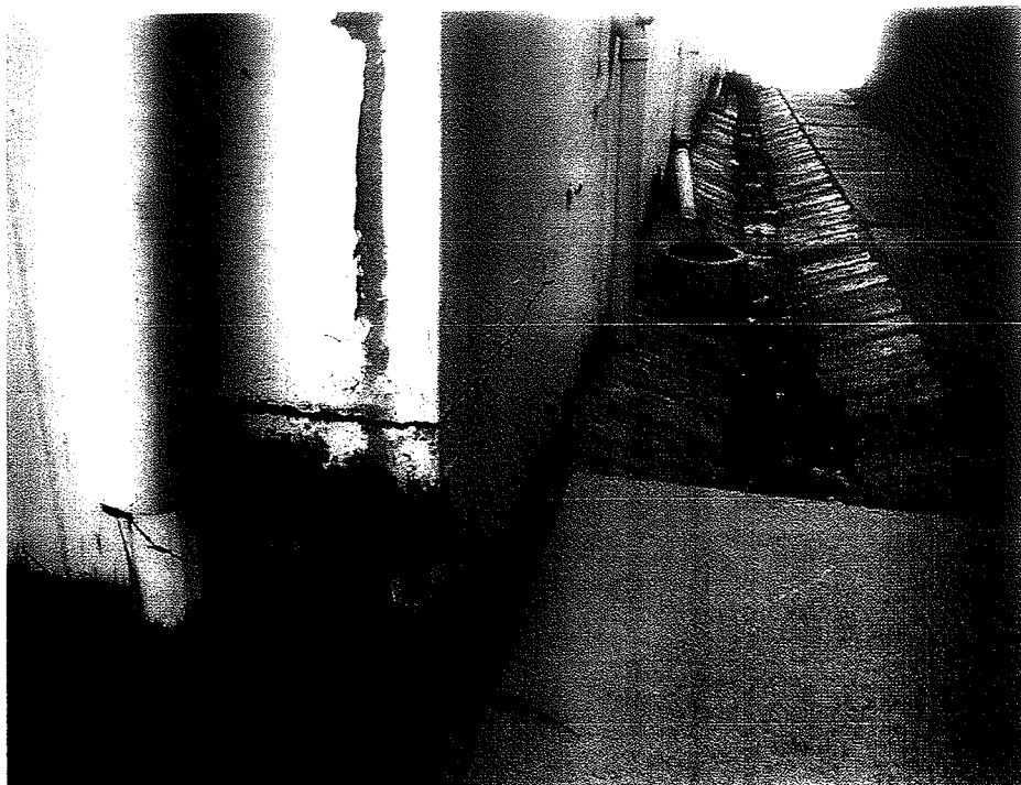
Photo 10 Detail at base of east corner of building showing downpipe discharging directly onto ground level and brick lined channel (not effective) around down pipe (Palassis Architects, July 2009).
