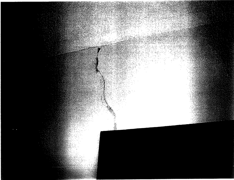
Photo 15 Detail of crack in north-west wall of waiting room (Palassis Architects, July 2009).
