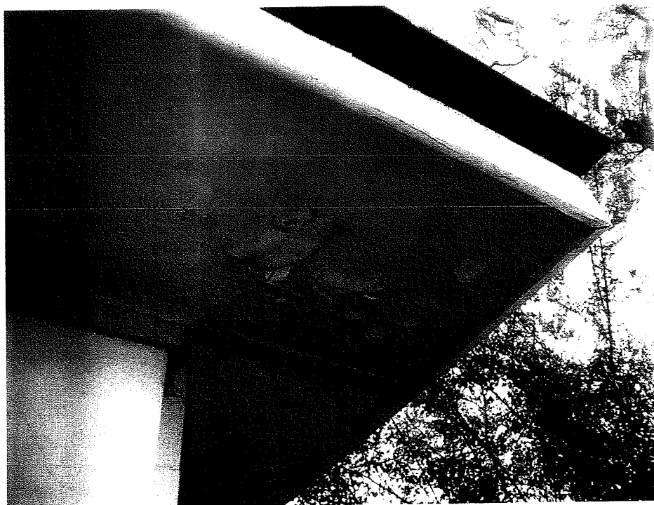
Photo 8 Detail of deteriorated and water damaged external paint finish to cementitious sheet eaves lining (Palassis Architects, July 2009).
