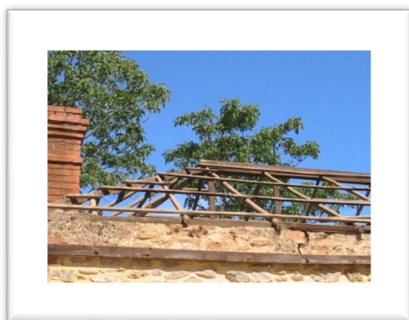
Exposed rafters during renovations
