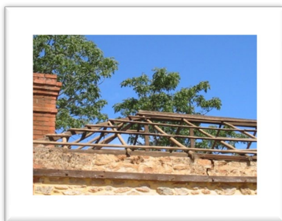
Exposed rafters during renovations
