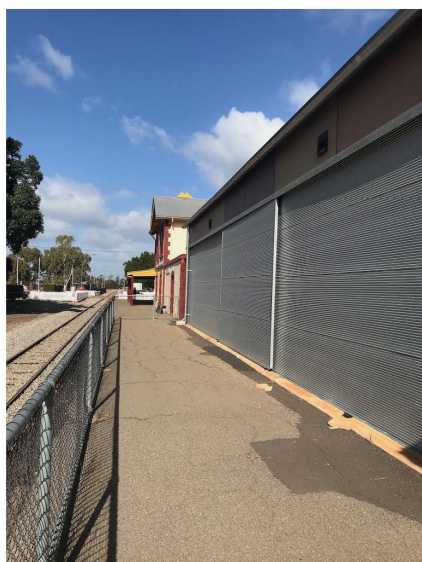
Views of the Platform Theatre looking south along the west side, and the east side that shows the proposed platform at the end on the left.
