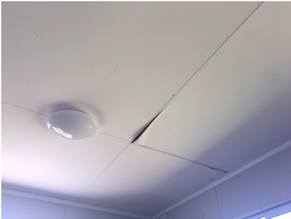
Minor water damage (top and bottom photos)
