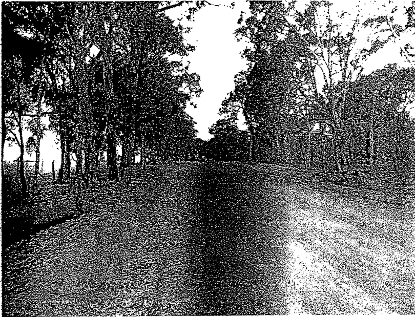
Figure 7. Edison Mill Road / Access to Lot 28061 - Sight Distance looking East
