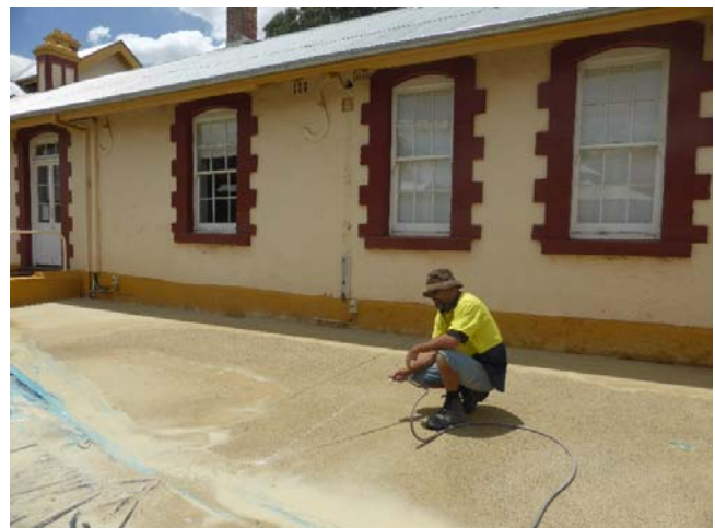
Rob Higginson hosing down the aggregate concrete
