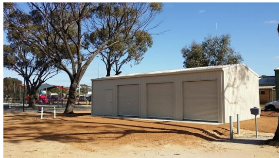
Equipment Storage Shed
